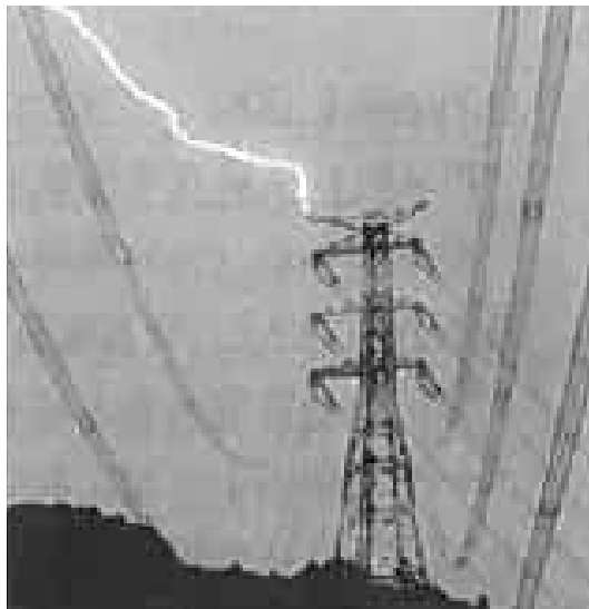
Lightning stroke to Grounding wire
